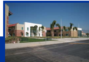
Jurupa Hills High School Construction completed on the over 265,000 square foot high school. The school will open at the start of the 2010-11 school year.
